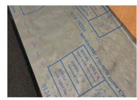
2 Mark the Centre Line: Once the roof is battened to match the panel profile, mark the centre line at several points along the hip.
