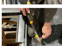
15 Adjust the Downturn: Where the flashing kit raises near the skirting, adjust the tile panel downturn to prevent it from sitting too high.
