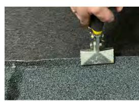
**3** Fit the Tile Panel: Position the prepared tile panel in the desired area and check the fit. If adjustments are needed, repeat the process.
