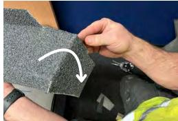
10 Close the End Cap: Fold the triangular flap on the inside of the flashing backwards to close off the end cap.
