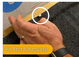
3 Lay the Panels in Broken Bond: Lay the panels in a broken bond pattern. Start by laying three courses, then secure the second course to the top course. Continue laying and securing the panels in this manner.
