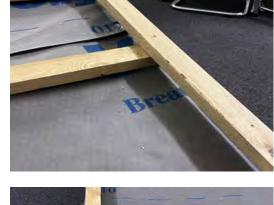
3 Extend the Verge Batten at the Eave: Ensure the verge batten extends 40mm beyond the fascia line at the eave.
