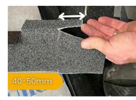
8 Fold the Outside Flap: Leave approximately 40-50mm of the outside flap. Fold it inwards at a 90° angle.
