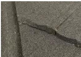
3 Secure the Panels: Once the courses are complete, secure the panels. Since the profile has been flattened to accommodate the downturn, place the first fixing point approximately 100mm from the bend line.
