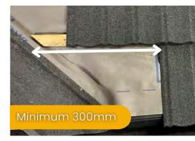
2 Start from the Top: Begin installing the panels from the top of the roof. Secure the first full tile panel to the batten nearest to the ridge battens using a tile nail, clout nail, or screw, being careful not to penetrate the membrane below.
