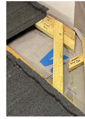
**3** Mark and Prepare the Tile Panel: Transfer the measurements to the tile panel, marking the bend line along with the top and bottom lines.
