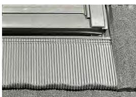
**20**Minimizing Tile Rise: Due to the design of granulated tile panels, there may be a slight rise near the rooflight. This can be minimized by carefully following the installation guide.
