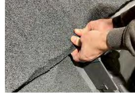
**Note:** If necessary, cut and fold the top tile panel like the side panels based on how the courses align.
