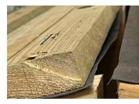
2 Install the Second Ridge Batten: Place a second ridge batten below the first one and secure it to the rafters. This provides a platform for the final tile panel to rest on.
