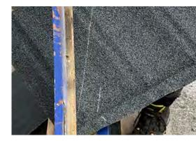
4 Make Final Adjustments: The cut should be even along the line, but if it's slightly off, trim any excess using the guillotine or snips.
