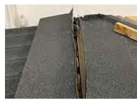
3 Measure and Secure the Ridge Battens: Measure and secure the ridge battens 100mm on either side of the ridge line.
