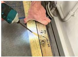
3 Repeat on the Opposite Side: Follow the same steps to install ridge battens on the other side of the ridge. Ensure there is approximately a 20mm gap between the battens on both sides to allow for proper airflow.
