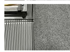
16 Flatten Tile Panels at the Skirting: Flatten the tile panels where they meet the side flashing.
