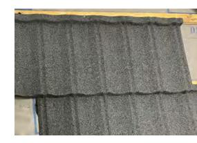
4 Walking on the Panels: Panels can be walked on, but ensure your heel or toe is on the batten and in the low area of the panel profile to avoid damage.
