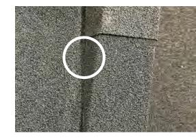
4 Secure the Verge Flashing: Use 3 fixings to secure the top of the verge flashing to the verge batten and 3 fixings through the downturn into the barge fascia. For overlapping flashings, ensure the lap is also securely fixed.
