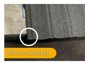
2 Secure the Eave Course: Secure the eave course at the top like the other panels, then fix it vertically into the eave batten below.
